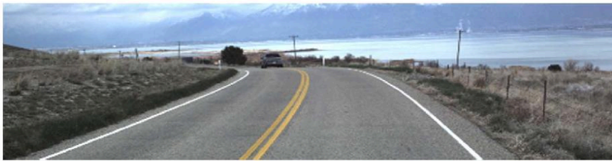
Figure 1: Roadway curvature without chevron markings (taken from Roadview Explorer 2014 image).
